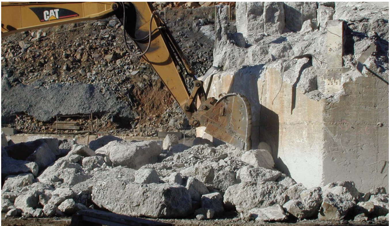
Breaking the concrete into 1/2 yard cubes made it easier to remove.
