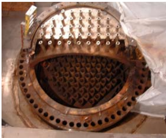
A partially segmented reactor head at Rancho Seco in Sacramento, California.
