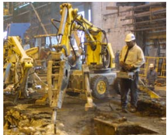
Rolling mill upgrade Nucor, Nebraska.
