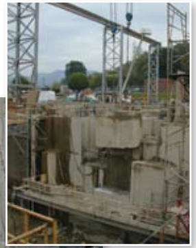
Rehabilitation project with mass concrete removal at London Lock and Dam on the Kanawha River in West Virginia.
