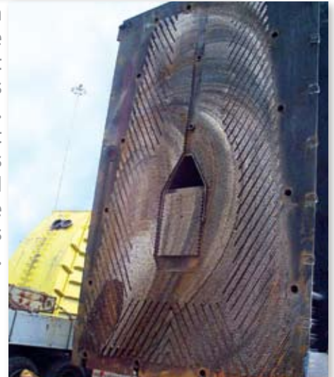
Two 120-ton condensers were split in half so that (4) 60 ton sections could be removed. The diamond wire cut through 27,000 tubes of inconel, 1/4" steel ducts and steel baffle plates. One cut was made in twelve hours.
