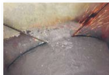
Nozzle cut at completion. Average cutting time for the six nozzles was 22 hours. No water or other liquid coolants were used. This minimized waste, and simplified the cleanup process.
