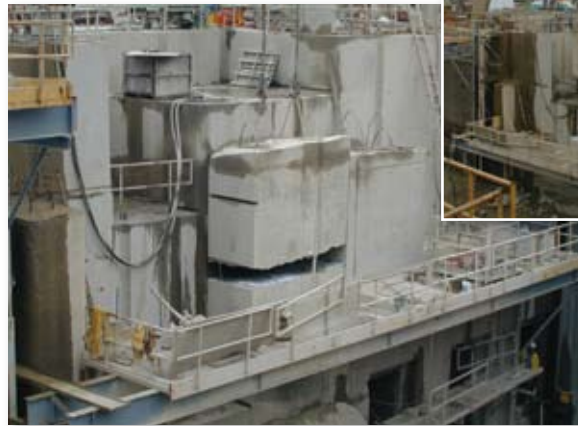
Two 120-ton condensers were split in half so that (4) 60 ton sections could be removed. The diamond wire cut through 27,000 tubes of inconel, 1/4" steel ducts and steel baffle plates. One cut was made in twelve hours.
