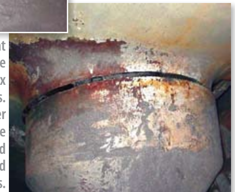
Reactor Nozzle Cut San Onofre, CA
