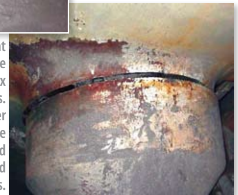
Reactor Nozzle Cut San Onofre, CA
