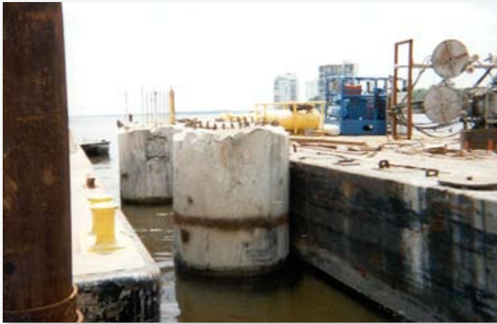
UNDERWATER CAISSON CUTTING, REMOVAL AND SMOOTH CUT CONCRETE FINISH.
