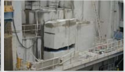
PLUG REMOVAL AT TALLULAH FALLS HYDROELECTRIC DAM
