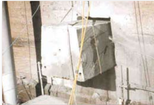
PLUG REMOVAL AT TALLULAH FALLS HYDROELECTRIC DAM
