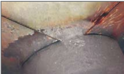
Fig. 1. Nozzle cutting in progress.
