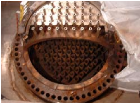
Fig. 6. An 8" thick steel reactor head segmentation by diamond wire saw.
