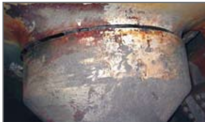
Fig. 2. Fully segmented nozzle after diamond wire sawing is complete.
