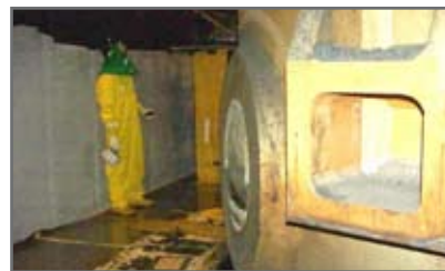
Fig. 10. Nozzle cut close to vessel surface to fit in canister.
