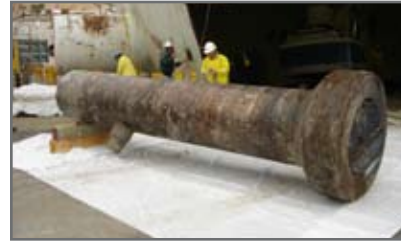
Fig. 8. Nozzle and safe end cuts made by diamond wire saw.
