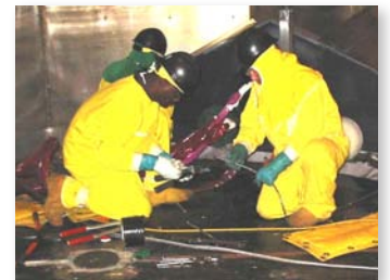
Reactor Nozzle Cut San Onofre, CA
