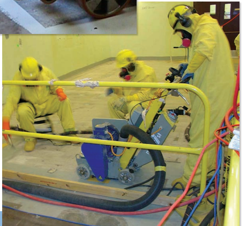
Left: Floor shaver removes coated concrete surface during technical demonstration at Argonne National Lab. Below: Floor shaver removes contaminated concrete for ease of surveying/monitoring during decommissioning of Building 371 at Rocky Flats Nuclear Weapons Plant.
