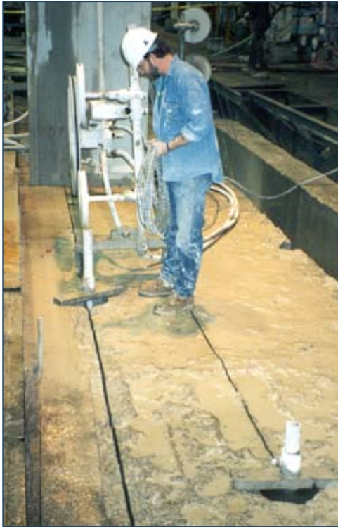
A wire being changed out during down hole wire sawing.
