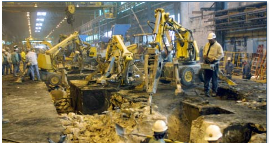
Rehab of the Nucor Nebraska II roll line.
